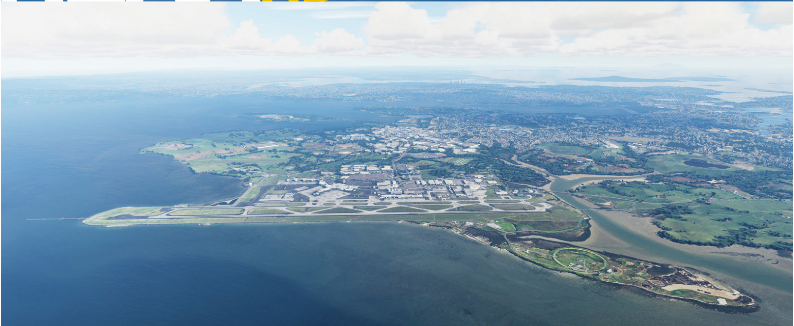
Auckland International Airport
